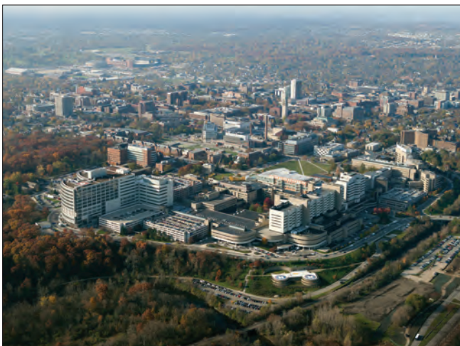
Aerial of the Medical Campus
