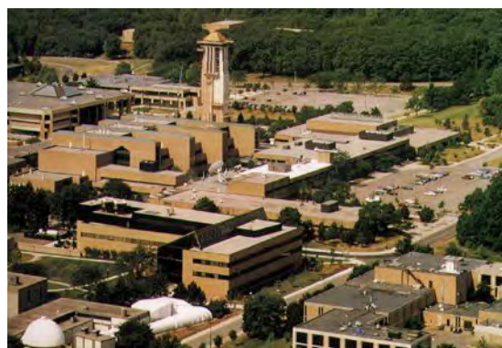
The completed North Campus
