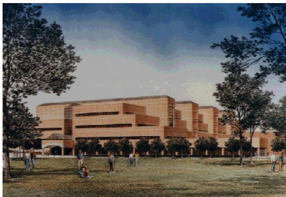
The new EECS complex
