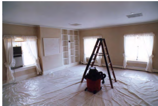
Stripping all the color from the house
