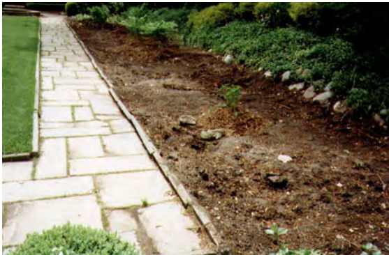
Digging out the old gardens
