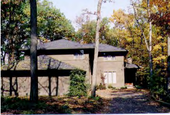
The house is ready
