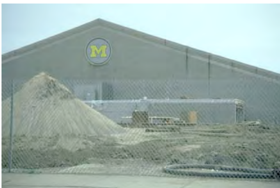
Surprise! The old locker rooms are gone!
