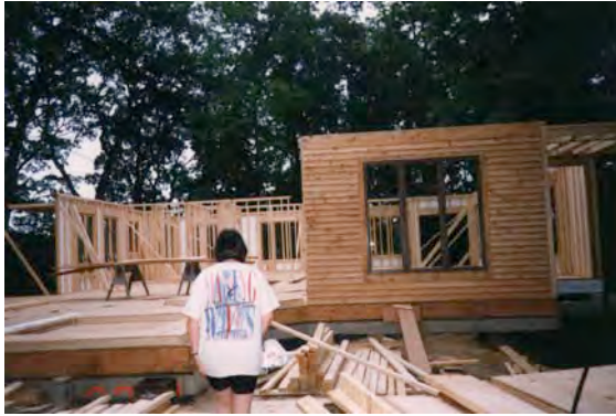
Early framing of the new house
