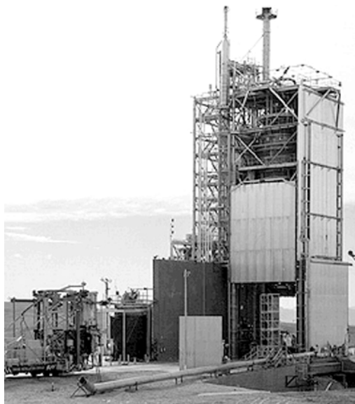
The Kiwi nuclear reactor test stand
